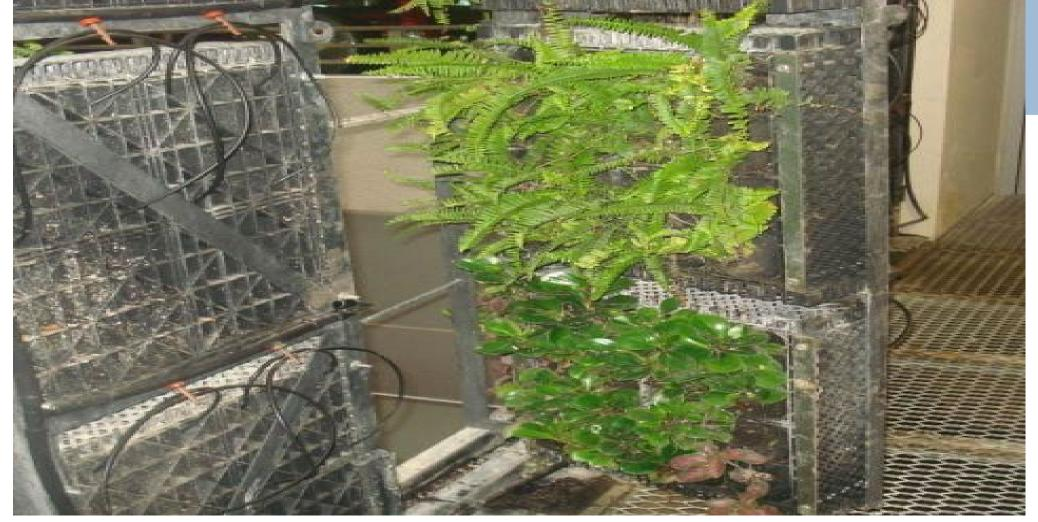
"French doors" allow the greenery to come to the worker. The camouflaged guardrail is aesthetically pleasing and is a passive control that allows workers to safely maintain and replace the 2023 State Construction Conference vegetation without much planning.
