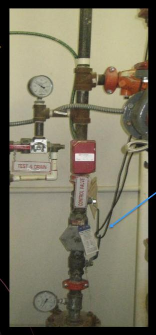
Tamper indicator using a "breakable cable type" Supervisory Switch.
