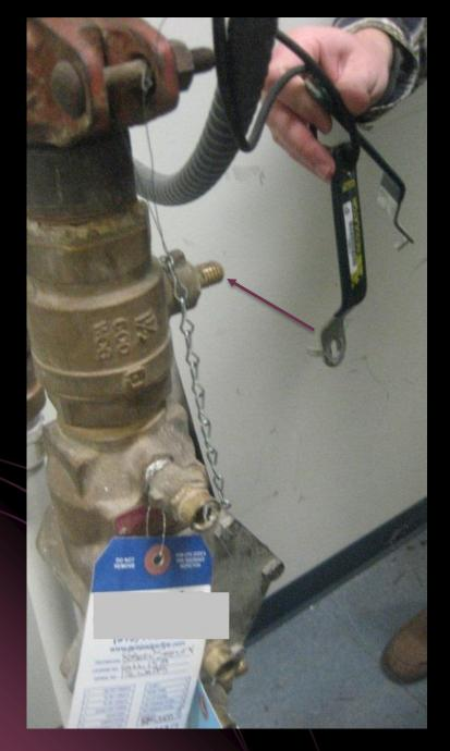
To eliminate breaking & replacing the electronic cable, the handles were removed at annual testing.
